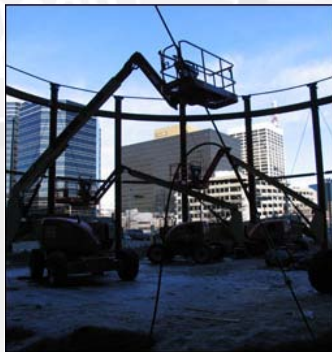
Prudential Center North/East Entry Cylinder Steel Framing
